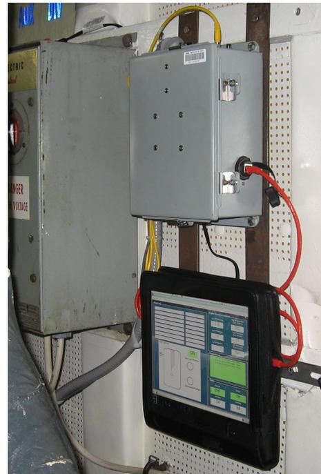
Fig. 5. NILM system as installed next to a power distribution panel on the USCGC ESCANABA. The NEMOmetrics sensor and data acquisition box, top, connects via Ethernet to a tablet PC, bottom.
